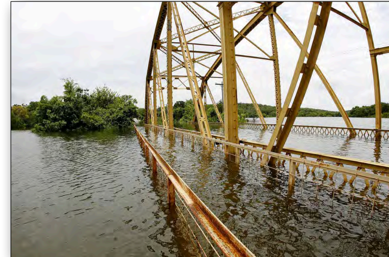
Rooster Creek Bridge, Lake Texoma, July 2007 (The Oklahoman)
